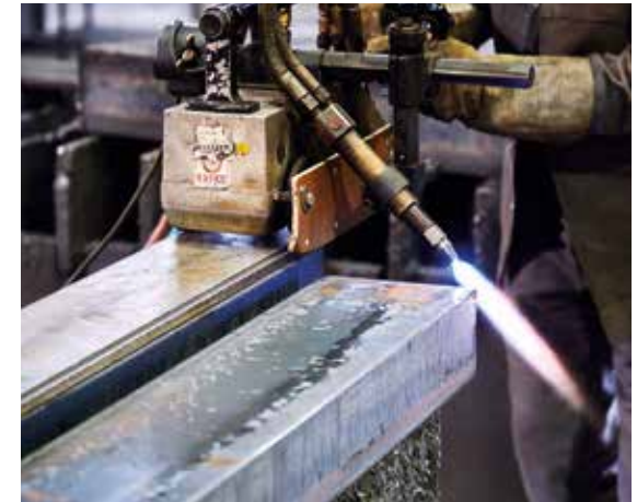
Thermal bevel cutting
