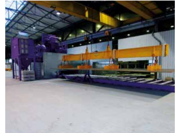
Loading the blasting machine
