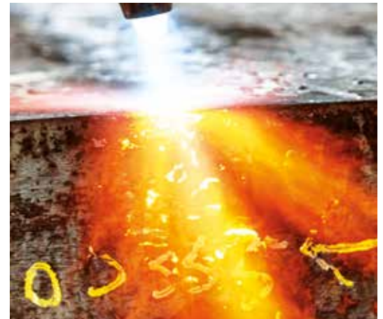
Flame straightening
